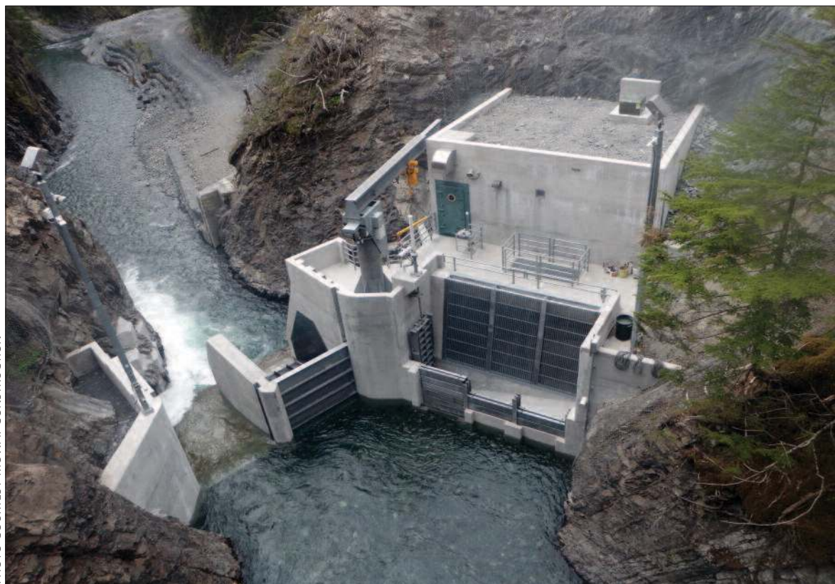
PHOTO COURTESY MOWAT CONSTRUCTION
