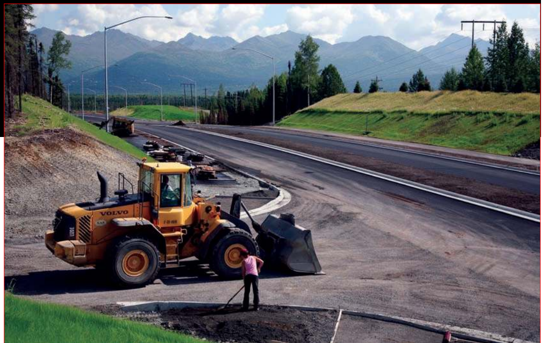
Dowling Road Extension, Anchorage
