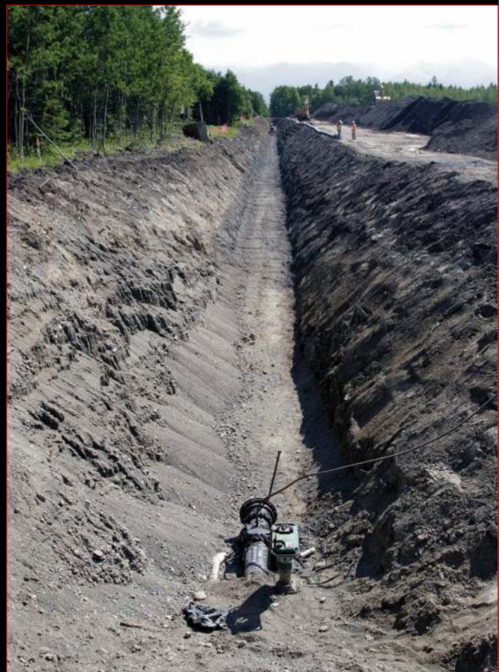
Sand Lake Water and Sewer Upgrades, Anchorage
