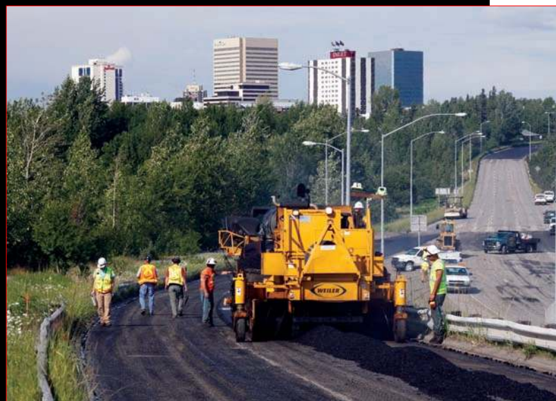
Minnesota Drive Resurfacing, Anchorage
