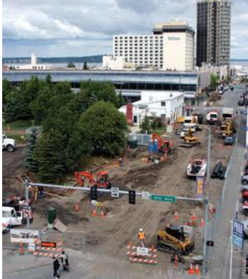
E Street Improvements, Anchorage
