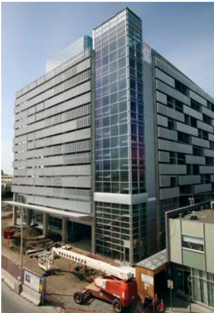
Linn Pacillo Parking Garage, Anchorage
