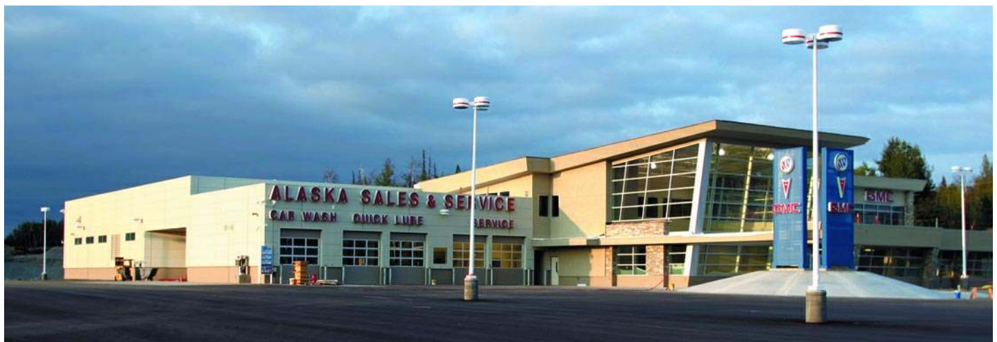
Alaska Sales and Service Building, Wasilla
