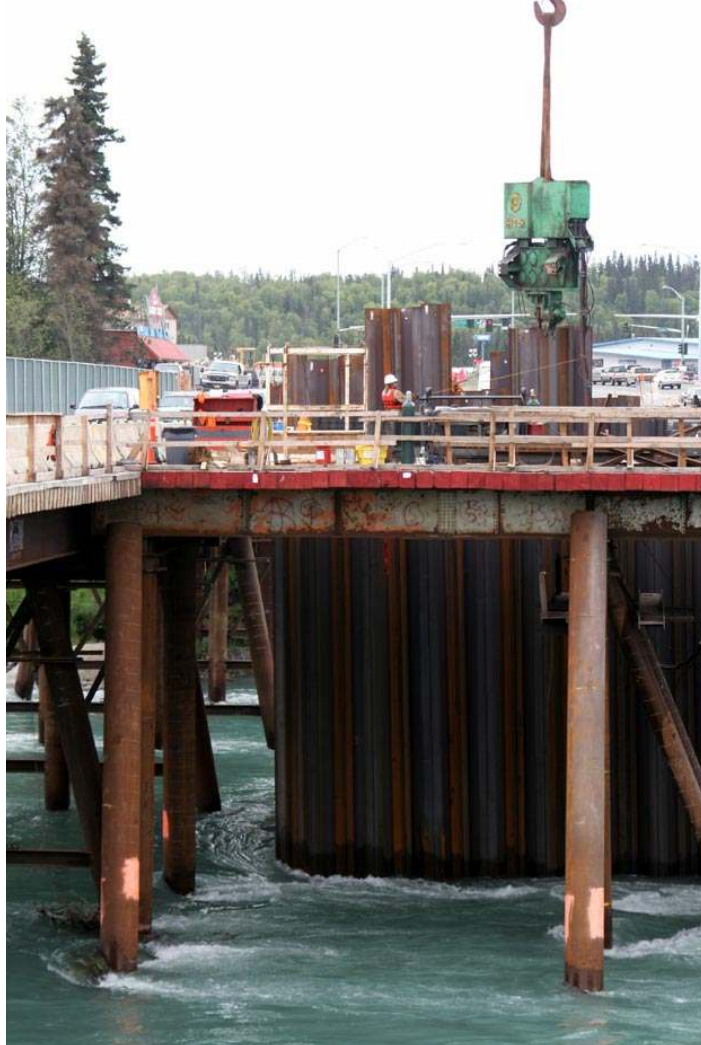
Sterling Highway Kenai River Bridge, Soldotna
