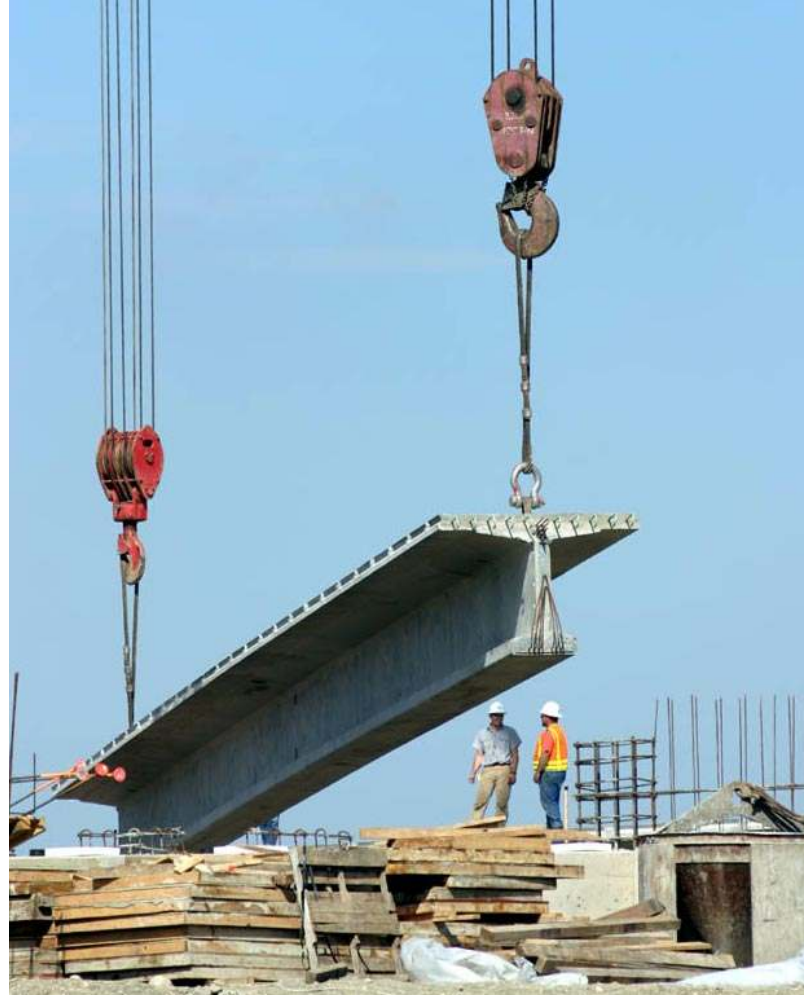
O'Malley Overpass/C Street Extension, Anchorage
