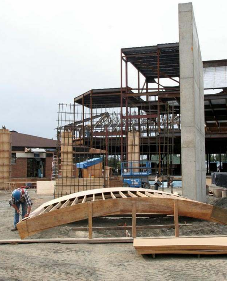
Central Peninsula Hospital Expansion, Soldotna
