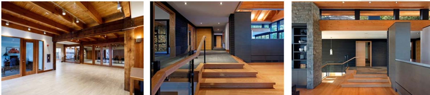
Interior Finishes: Exposed wood roof deck, painted drywall, commercial grade millwork
