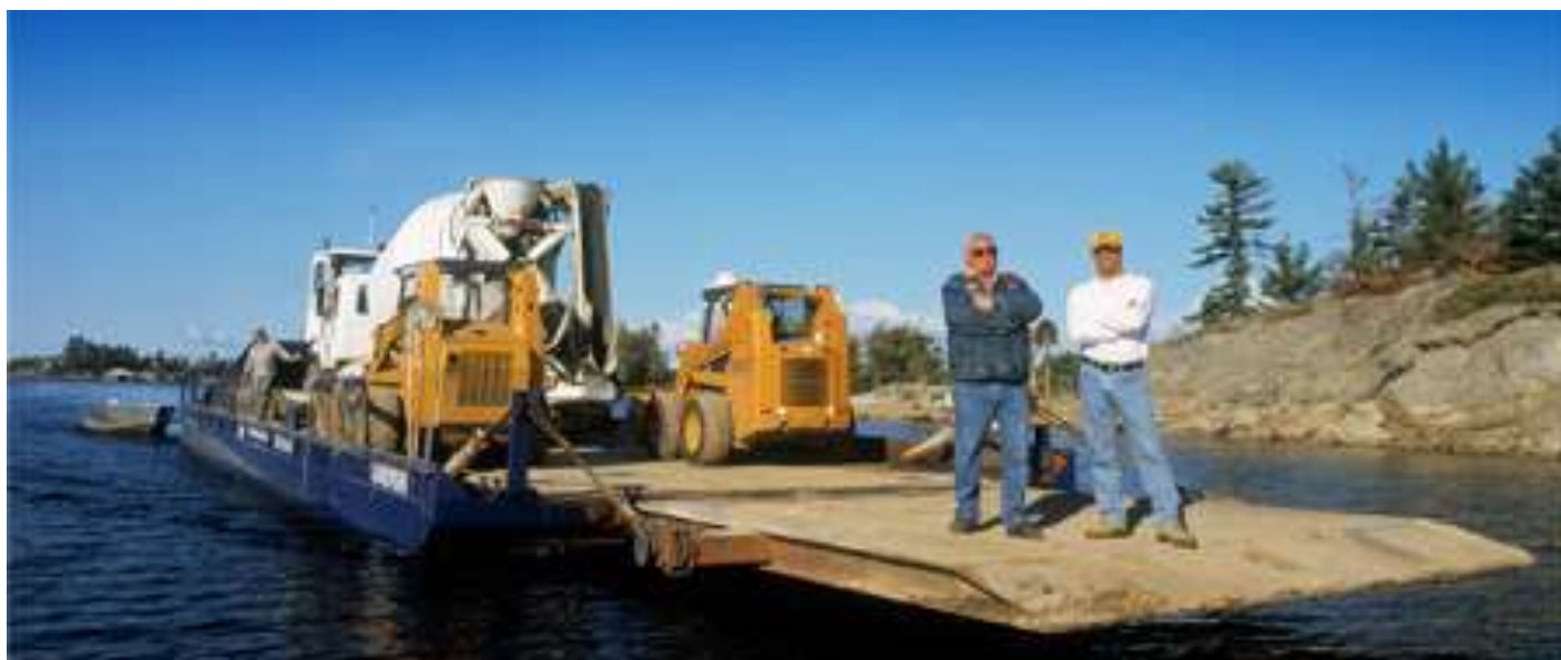
White Contracting & Barging
