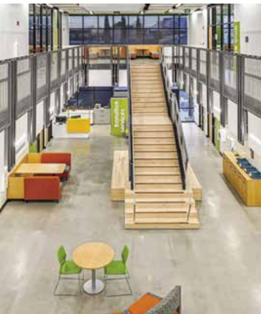
Part of Albuquerque Public Schools, the Lowell West Complex is a new 45,362-sq-ft, 2-story facility consisting of a combination of structural steel framing and structural masonry construction plus an approximately 3-acre site-development package.
