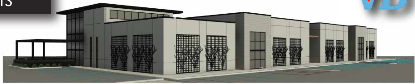
② PAD 6 REAR VIEW
