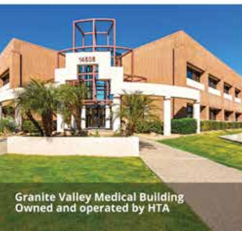
Granite Valley Medical Building Owned and operated by HTA
