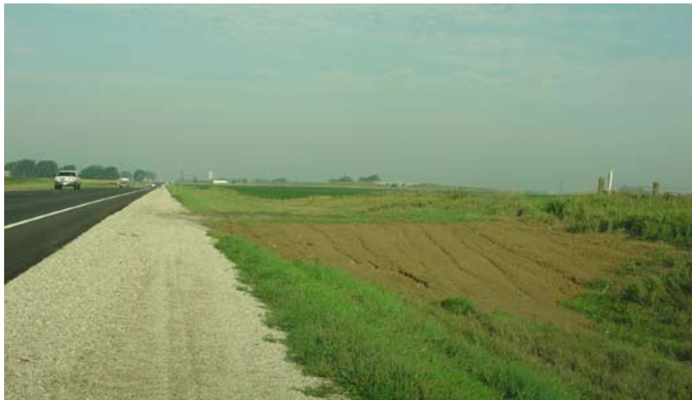
Figure 30. Farm field entrance slope flattening in Iowa. (Source: Courtesy of IADOT)
