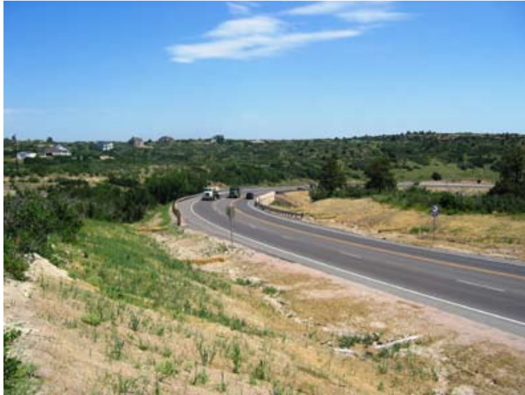
Figure 5. Upgrade climbing lane added with resurfacing in Colorado.
