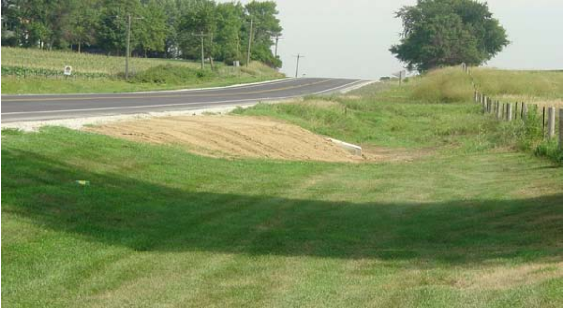
Figure 18. Culvert extension in Iowa. (Source: Courtesy of IADOT)
