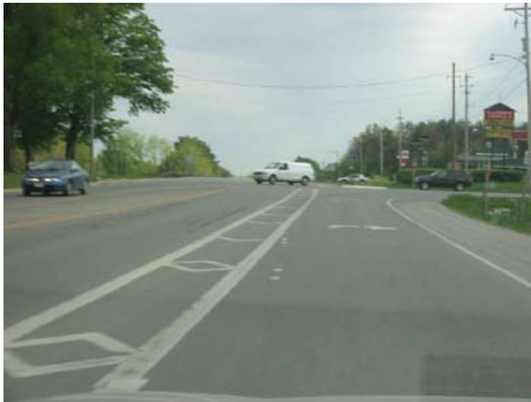
Figure 6. Addition of turning lane in Iowa. (Source: Courtesy of IADOT)
