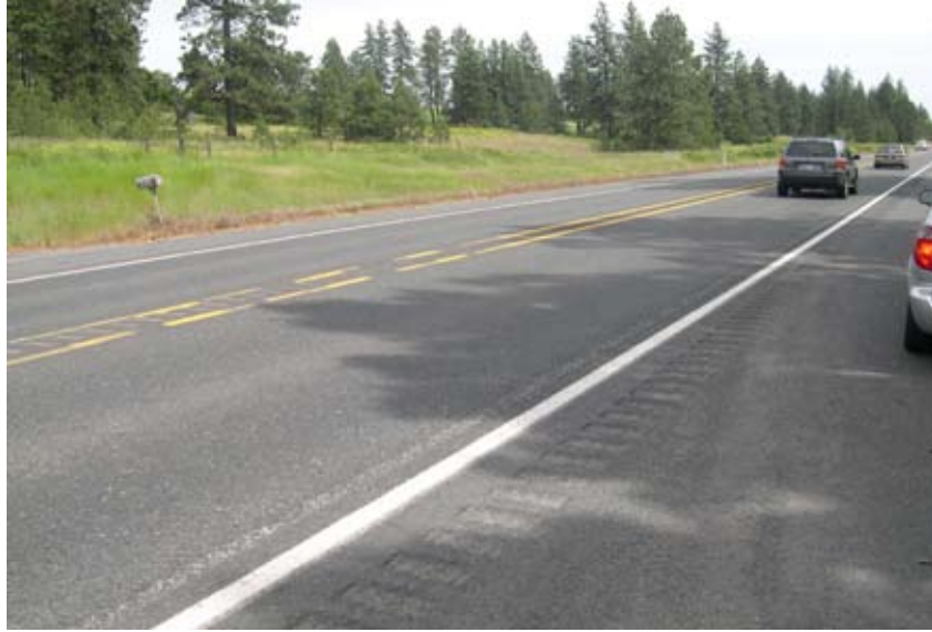
Figure 12. Centerline and edge rumble strips in Washington State.
