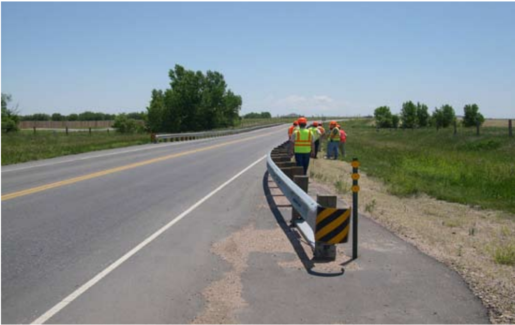
Figure 22. Guardrail terminal and pavement in Colorado.
