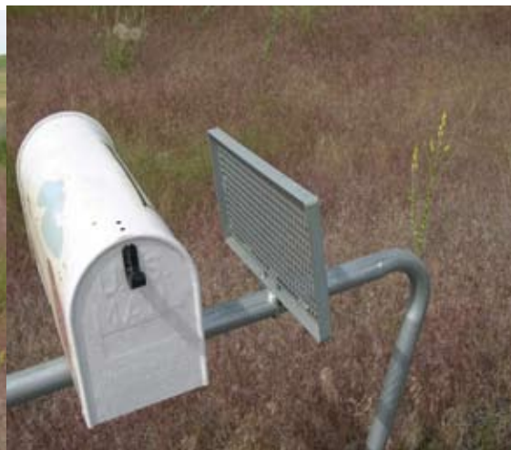
Figure 24. Close up of a crashworthy mailbox installation in Washington State.
