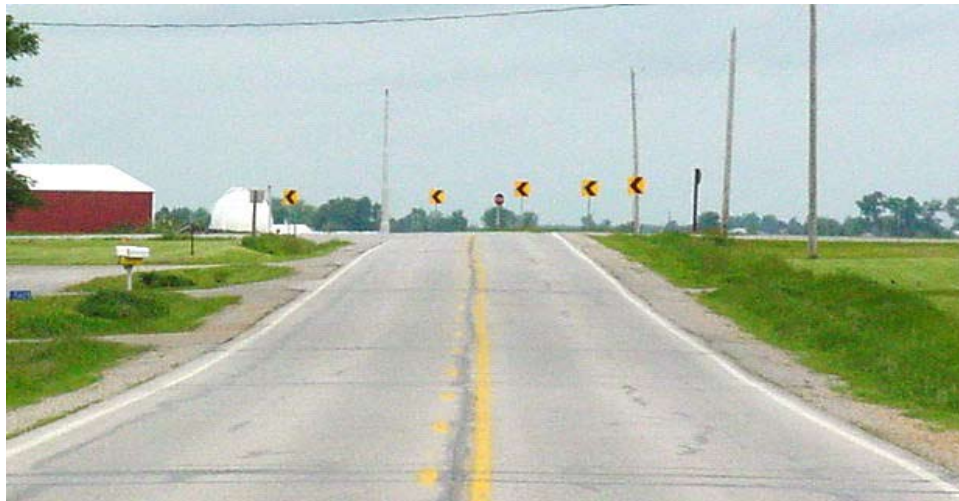
Figure 15. After placement of chevrons on horizontal curve in Iowa. (Source: Courtesy of IADOT)
