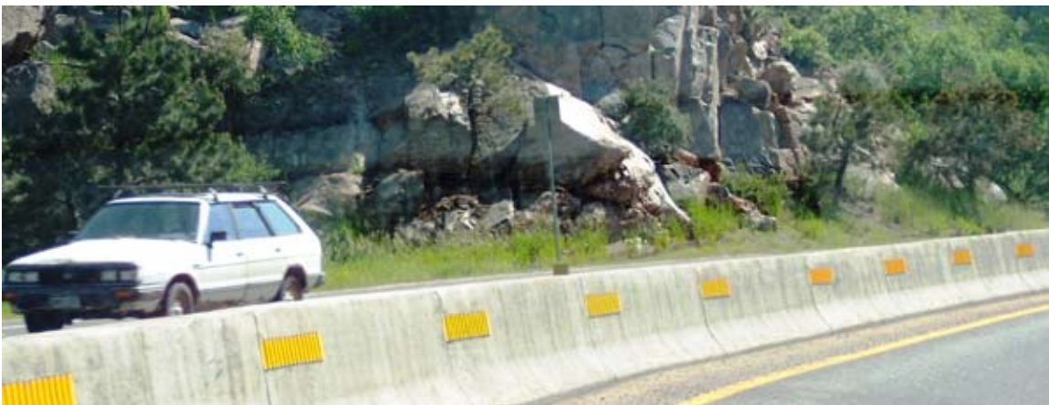
Figure 13. Sheet delineation on median barrier in Colorado.
