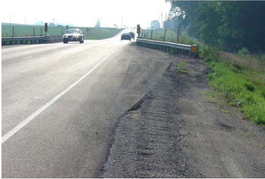
Figure 16. Bridge approach rail, Iowa. (Source: Courtesy of IADOT)
