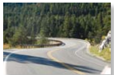
The cost of w-beam guardrail will vary regionally and over time. However, in-service studies reported a range of $11.44 per foot (2004) to $13.65 per foot (2003). 9,10 Adjusted to 2011 dollars, these figures would be $13.71 to $16.80, respectively. 11
