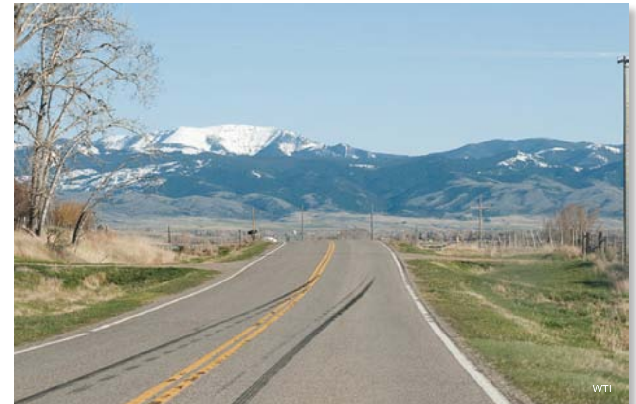
Visual indications, such as skid marks, can identify potential safety issues during a field audit.
