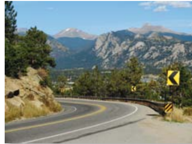
Chevrons improve curve delineation and provide warning of an alignment change. Photo by William Shorb.
