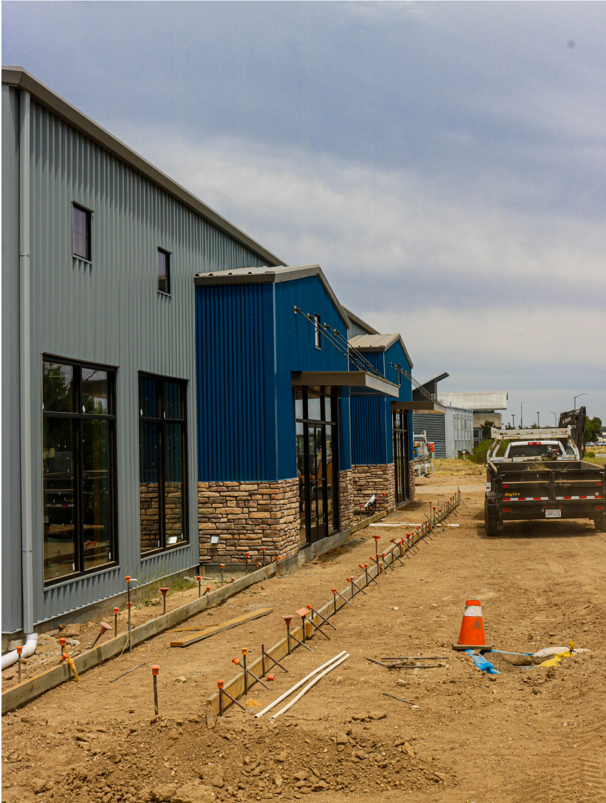
New building under construction on Dallons Drive.
