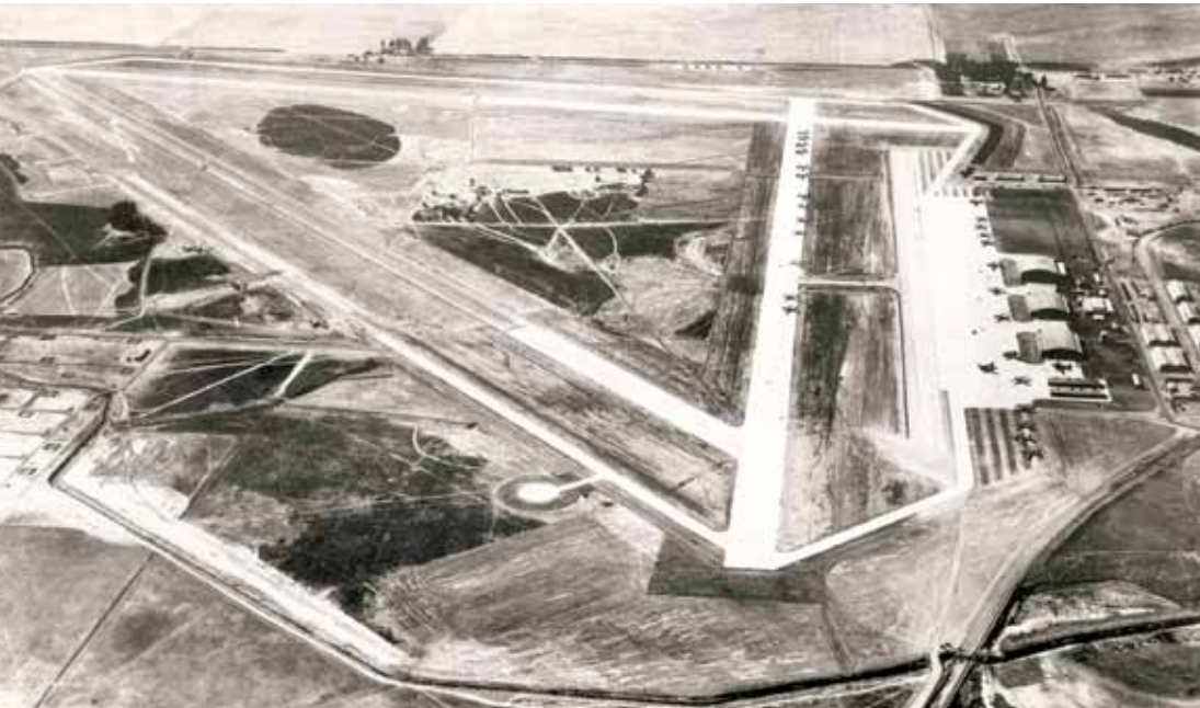
The runways were completed at Fairfield-Suisun Army Air Base on June 1, 1943. (USAF photos)
