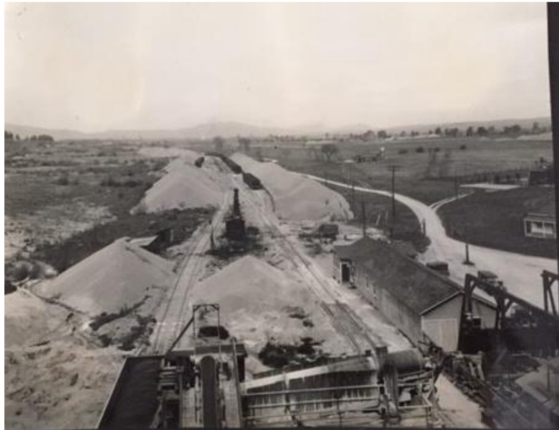
ENORMOUS STOCK PILES OF SAND, ROCK AND GRAVEL AT ONE OF OUR ELLIOT PLANTS (CALIFORNIA BUILDING MATERIAL COMPANY). THESE EXTENSIVE STOCK PILES ENABLE THIS PLANT TO SHIP 1,200 CARS PER MONTH.
