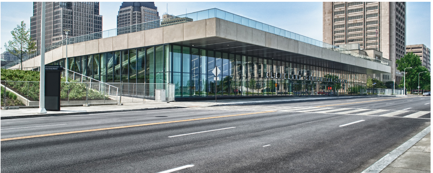
Cleveland Convention Center, Karpinski Engineering
