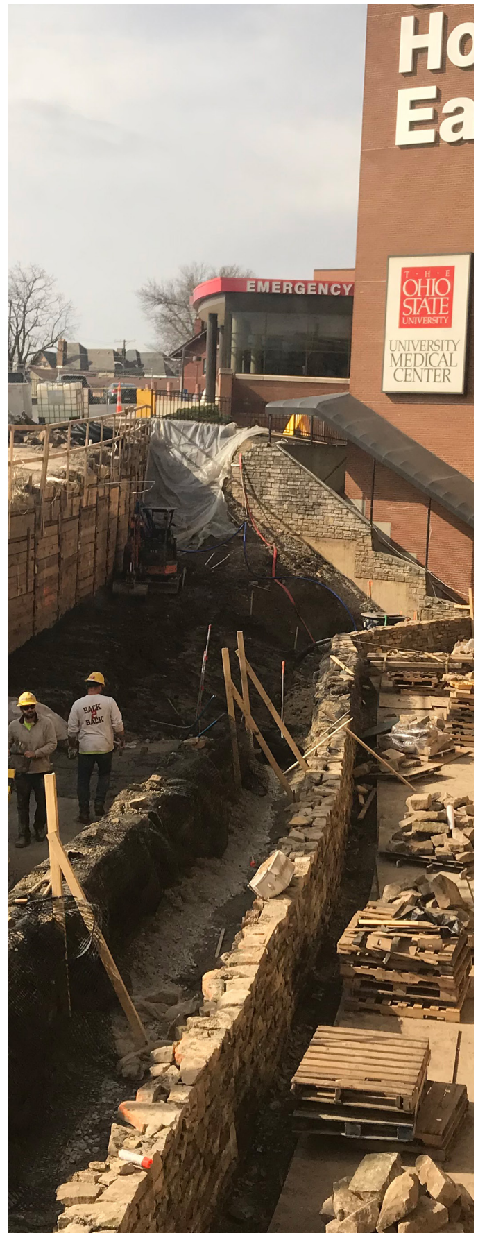
University Hospital East Courtyard Retaining Wall, Pennoni
