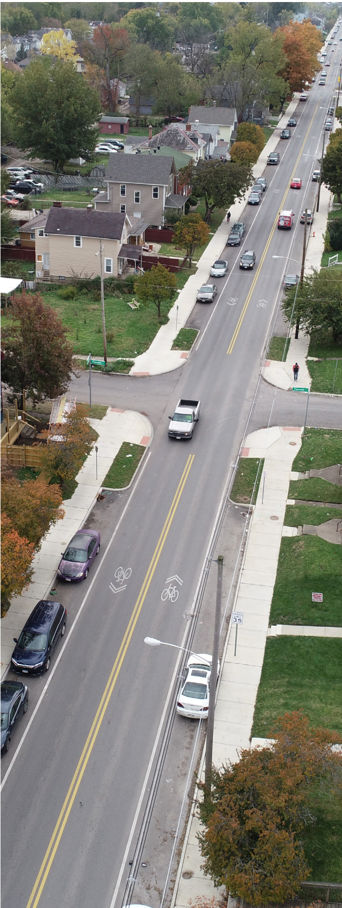
Hague Avenue Rehabilitation, Crawford, Murphy & Tilly
