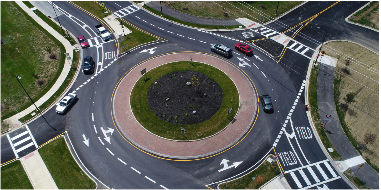
Hamilton Road Widening and Roundabout, ms consultants
