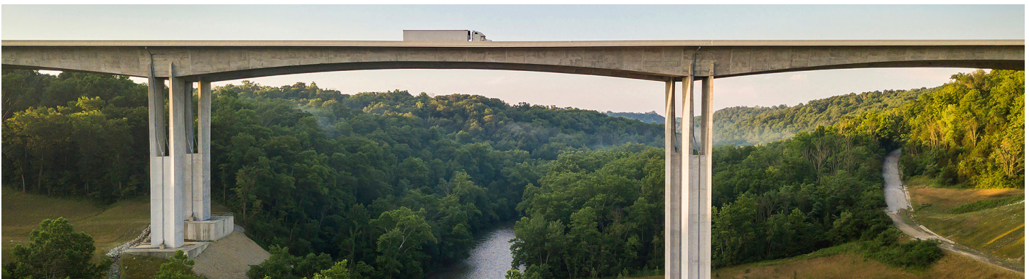
Jeremiah Morrow Bridge, HNTB
