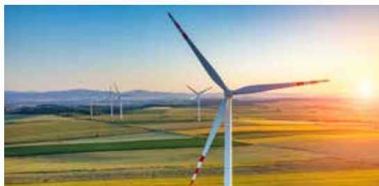
Fig. 15: Wind turbines - The fibre reinforced plastic (FRP) rotor blades are adhesively bonded.
