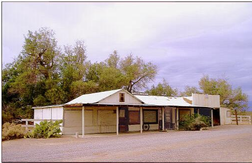
Borrego Springs' first store – built by Eslie Wynn in 1929 – Old Borego Town site
