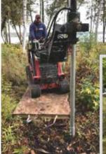
Helical Piers can be installed through wetlands for boardwalk and deck foundations. Beams are attached to brackets for traditional deck framing.
