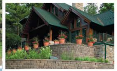
Keystone Retaining Walls
