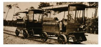
The standard-gauge Fellsmere Railroad was completed in 1910 with 60 lb. rail to replace the old Sebastian & Cincinnatus narrow-gauge railroad built between Sebastian & Fellsmere. The Fellsmere Farms Company used the 10 miles of railroad from September 1910 until May 1, 1911 for carrying logs to the Florida East Coast Railway in Sebastian and for transporting supplies, equipment, and heavy machinery used for excavating drain-age canals to Fellsmere.
