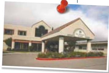
Newest addition of hospital completed
