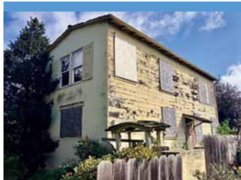
Blighted buildings in the City of Salinas.
