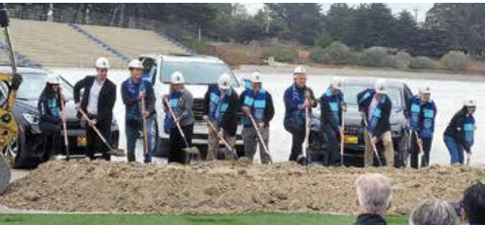
Groundbreaking for the new Cardinale Stadium for the Monterey Bay FC soccer team.
