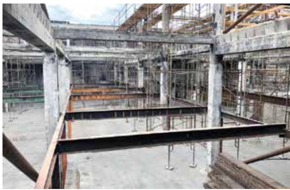
A peek inside the Bruhn Building construction.
