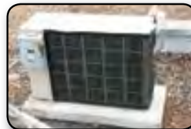
Air Cooled Condenser Intake Filter
