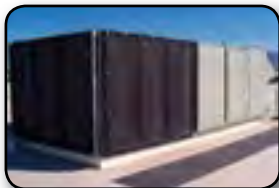
Rooftop Unit Intake Filters
