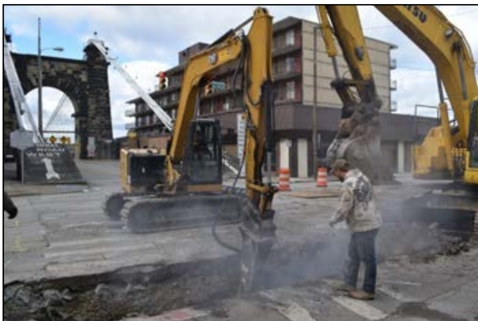
Crews with Pro Contracting Incorporated of Lost Creek work to install new waterlines throughout downtown Wheeling. The project includes replacing 20-inch water lines that are more than a century old with new 16-inch lines. The project is on schedule and is expected to be completed in February.
