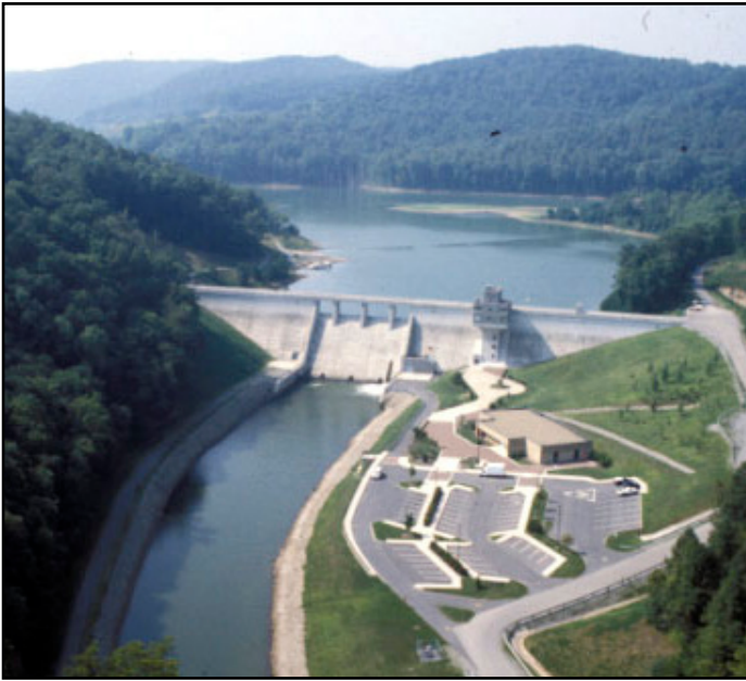
J.F. Allen Company (with joint venture partner Wiley N. Jackson Company of Roanoke, VA) built Stonewall Jackson Dam for the U.S. Army Corp of Engineers. After successful completion of the project, J.F. Allen Company was recognized by Engineering News Record as one of the “Top 100 Contractors” in North America.
