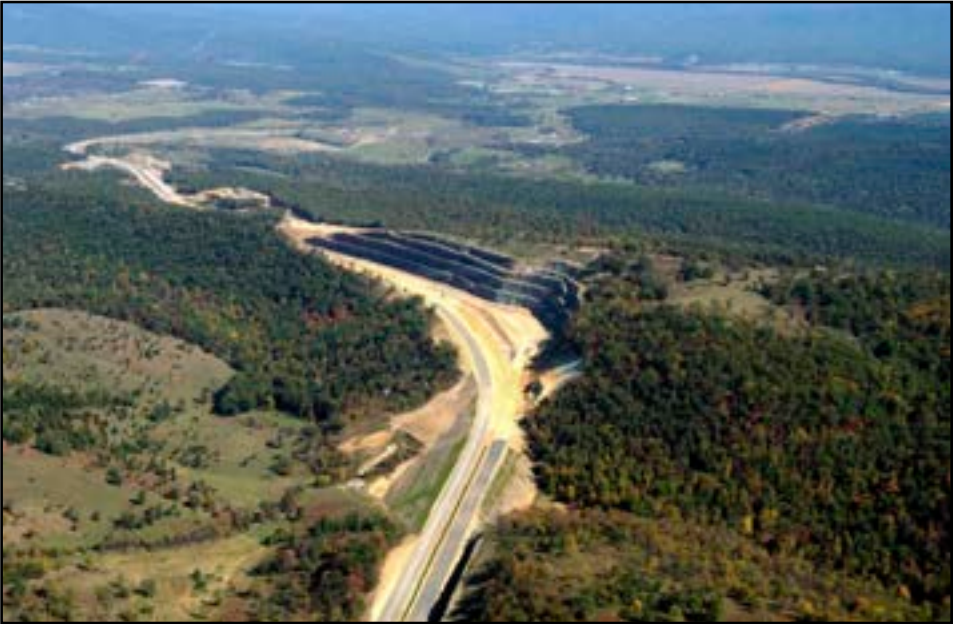
The company completed the remaining new highway section of Corridor H from Davis to Bismarck. This includes the moving of 2.7 million yards of dirt, 9.9 miles of new highway and 6.4 miles of new bike path. Upon completion of this project, J.F. Allen Company has now completed over 35 miles of construction in this important corridor.
