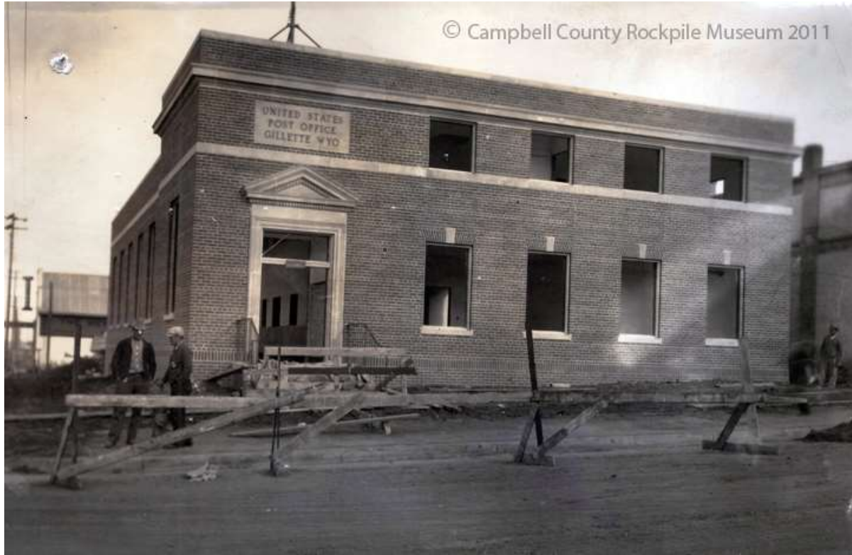
Gillette Post Office under construction in 1935
